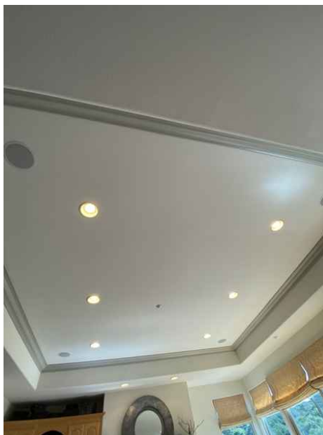
Ceilings: Ceiling Material Gypsum Board
